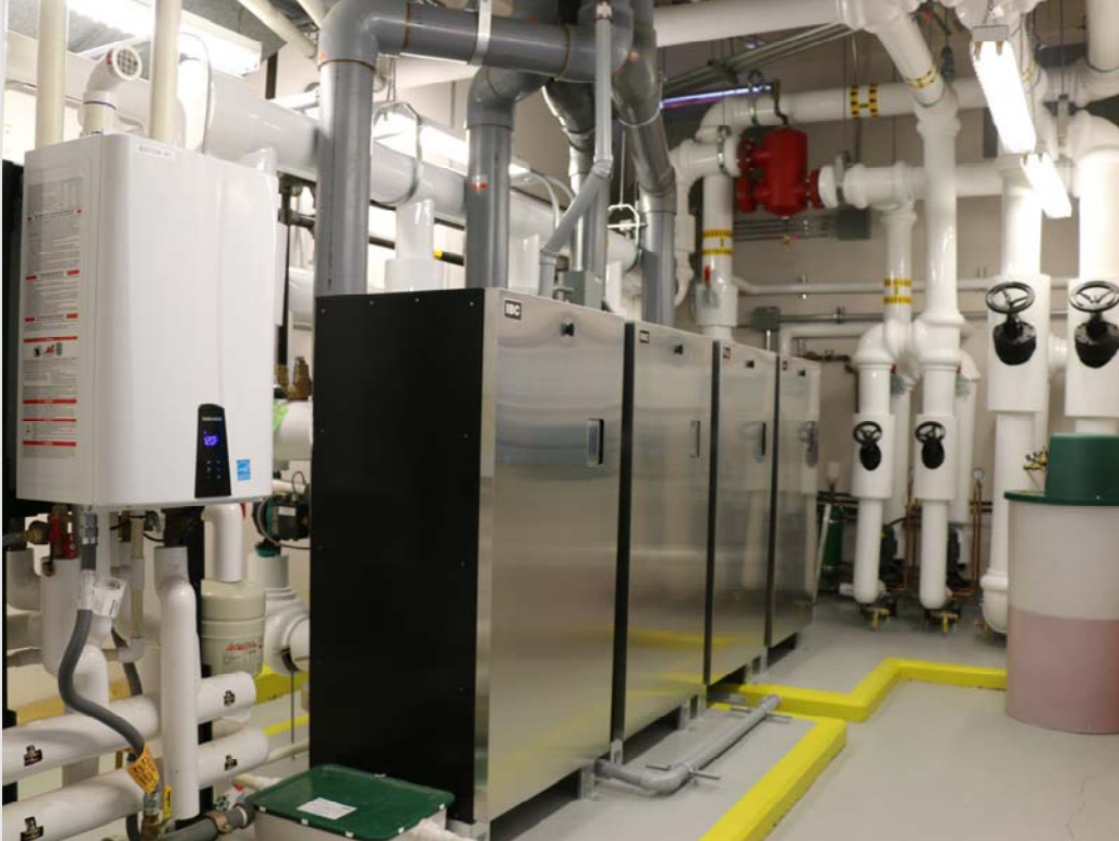
Heather Park Elementary—Boiler Replacement Summer 2022
