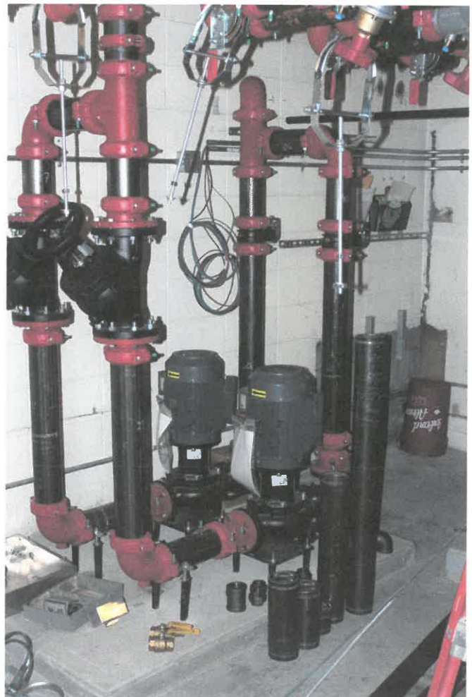
Buckhorn—System pumps being installed during construction.
