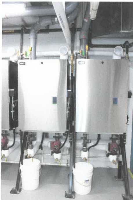
Buckhorn—System pumps being installed during construction.
