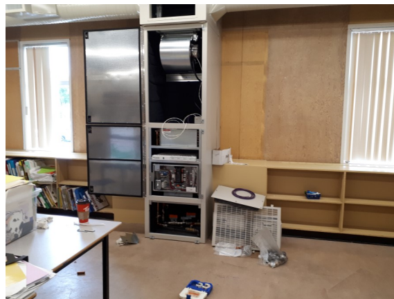
Apollo unit ventilators in each classroom—construction photo
